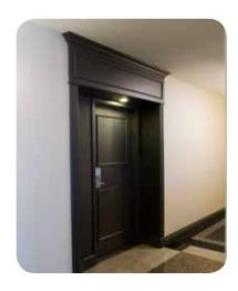
dark accent. The existing light lens at the elevator walk-off bulkhead was removed and pot lights were installed.
